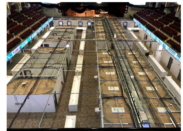
Interior Build Out
